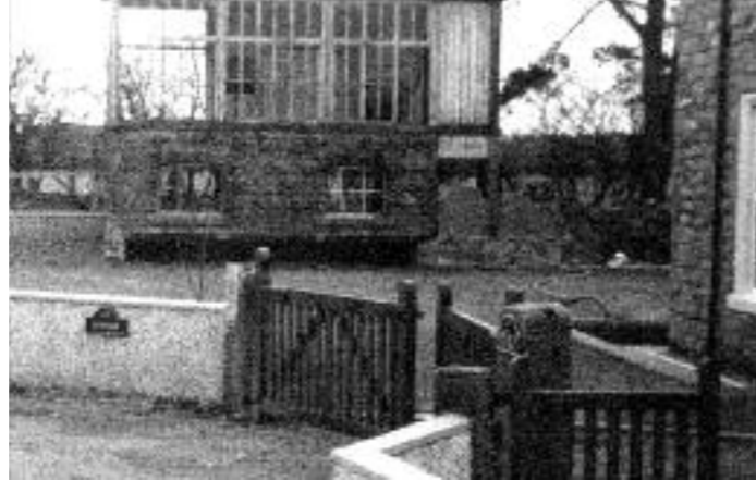
What remained of signal box on opposite side of track.
